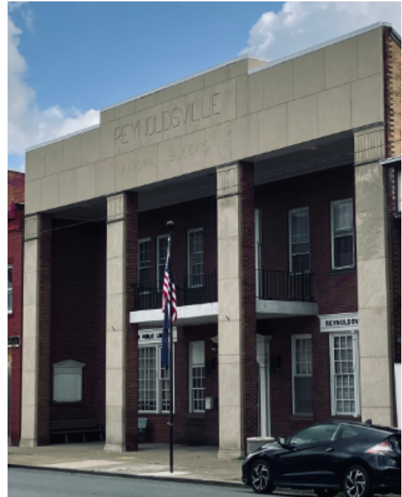
Borough of Reynoldsville Municipal Building Photo Courtesy: Borough of Reynoldsville
